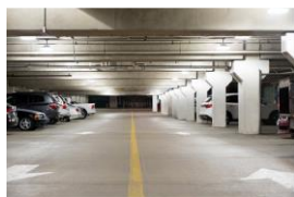
Figure 4. A parking structure that SOA formation experiments can be performed
